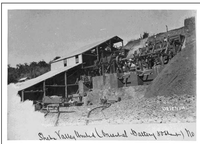
Figure 12. A 50 stamp battery erected to crush ore from the mines in the Sheba Valley. Other batteries were built on the Kaap River to the north, where the water supply was more regular.
